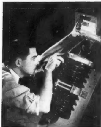
A breaker has been developed that allows reclosing to be applied on the smaller branch feeders of a distribution system.
